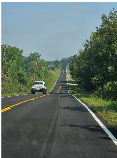
180 th Street after micro-surfacing and striping work.
